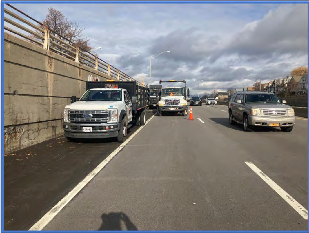
Photo 1 – Work Zone Traffic Control (WZTC) was conducted by U.S. Traffic Control.
