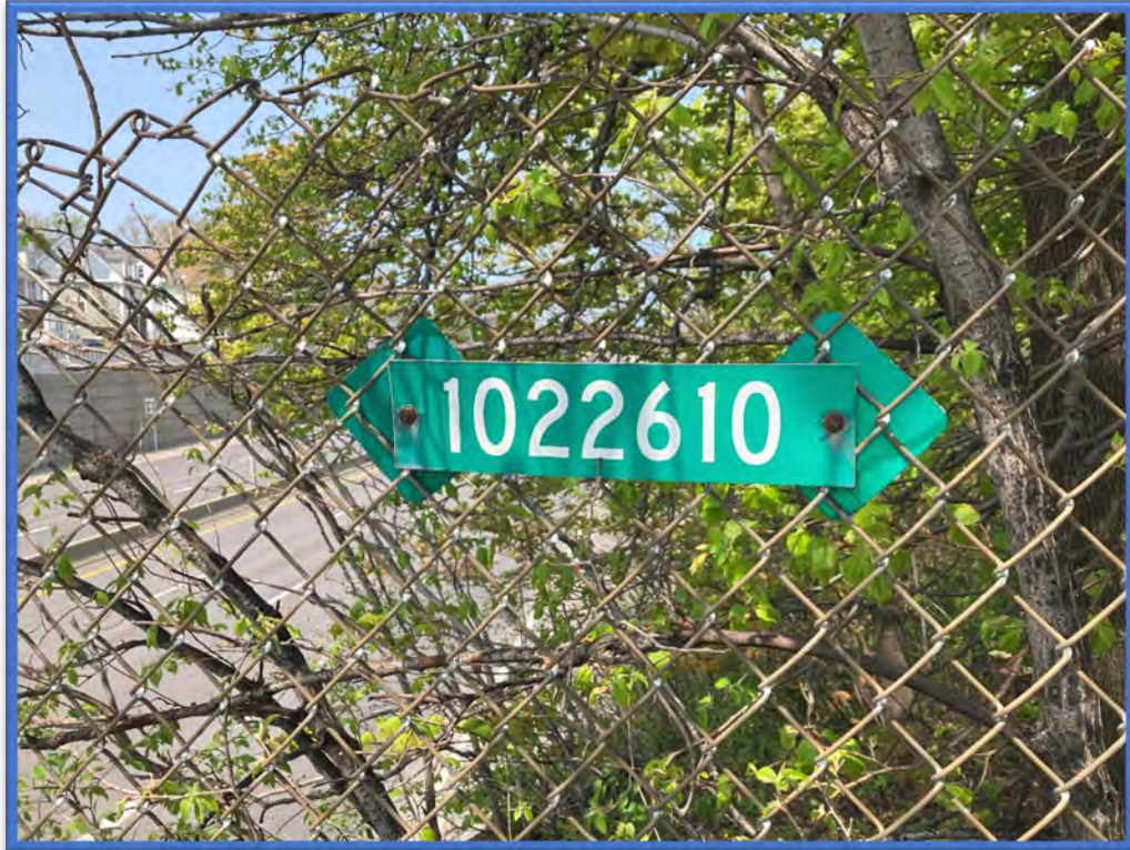
Photo 5 – View of the BIN plate located on the adjacent fence at the northeast quadrant of the Dodge Street Bridge over Kensington Expressway (Route 33) (BIN 1022610).
