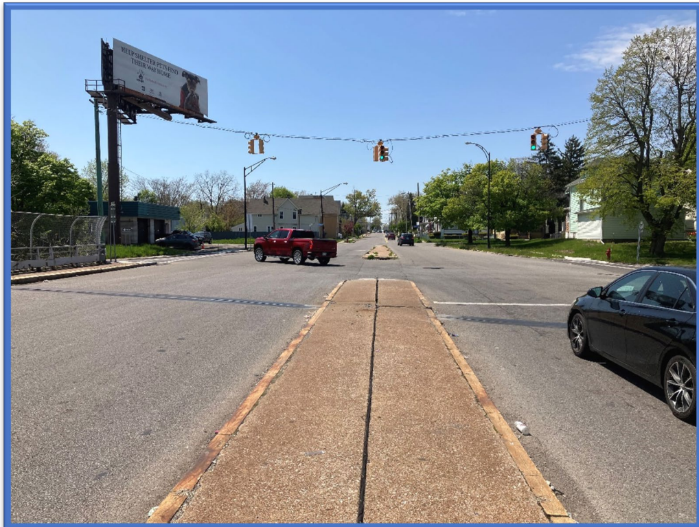
Photo 4 - View to the west from the middle of the E Utica St Bridge over Kensington Expressway (Route 33) (BIN 1022630).
