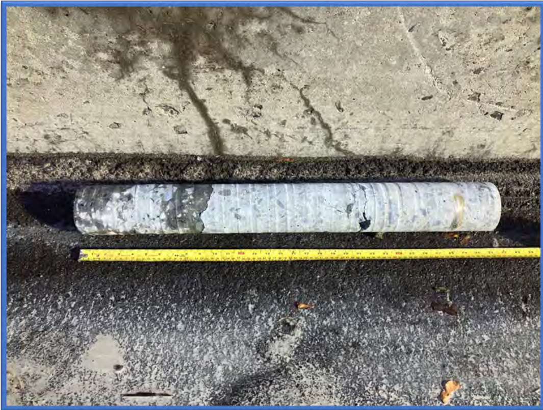
Photo 5 – Complete retaining wall core.
