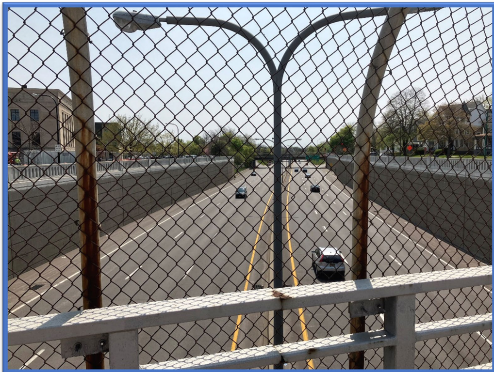
Photo 4 - View to the south from the middle of the deck of the Northampton Street Bridge over Kensington Expressway (Route 33) (BIN 1022620). Project corridor retaining walls are visible in the background of the photo. ACM caulking is only associated with the older lower portion of the walls.
