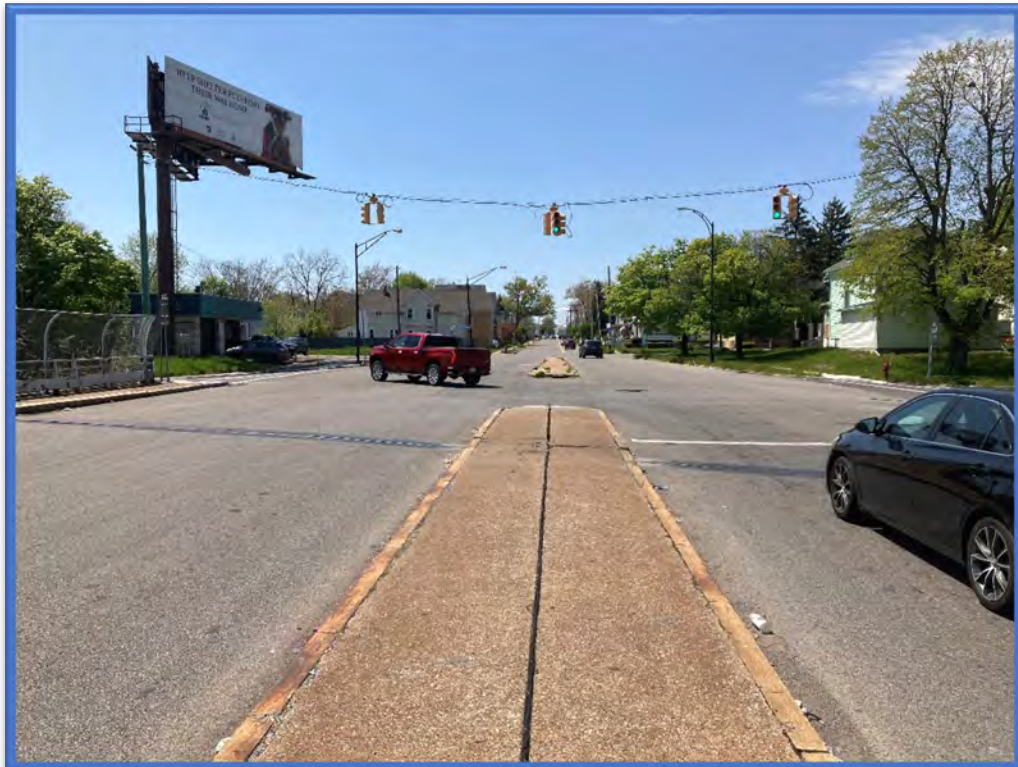
Photo 4 - View to the west from the middle of the Best Street Bridge over Kensington Expressway (Route 33) (BIN 1022609).
