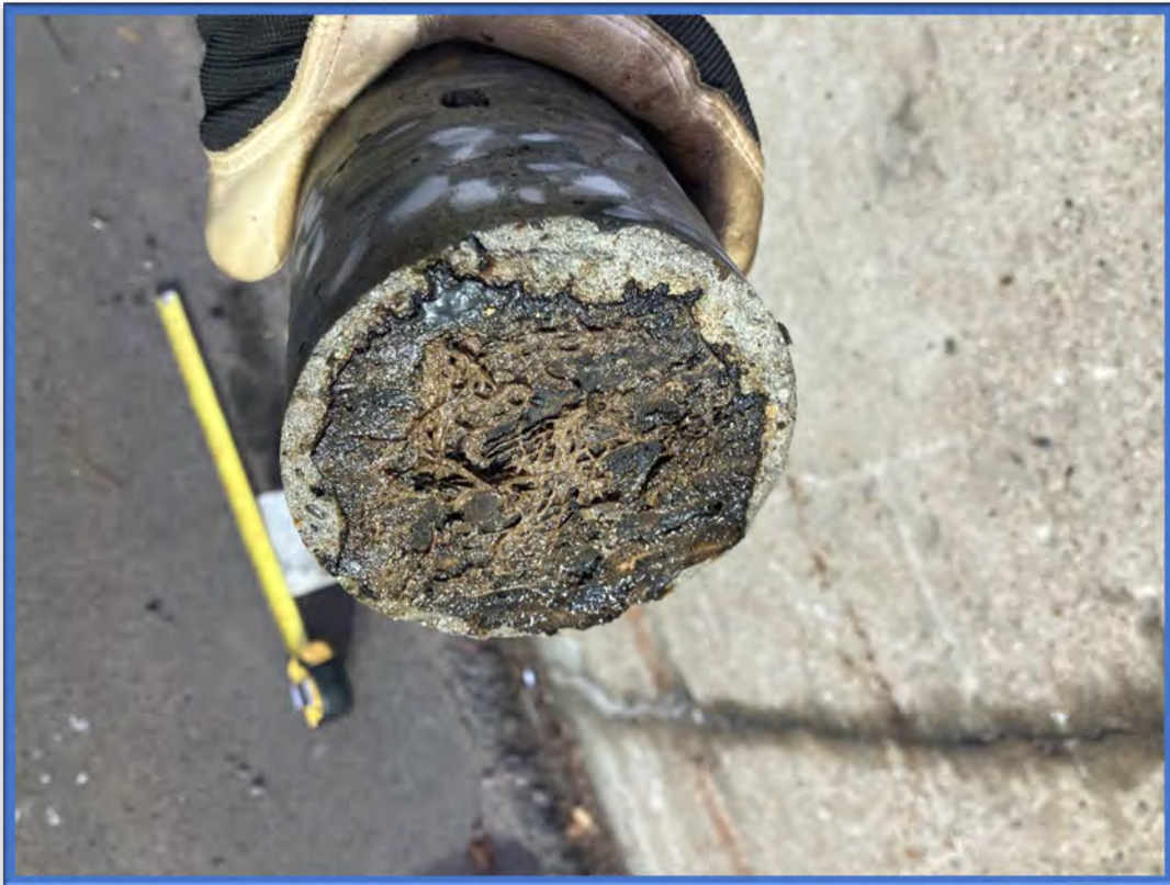
Photo 4 – Waterproofing tar located on the back of the retaining walls.
