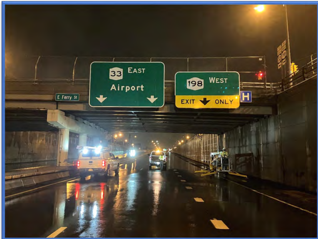
Photo 6 – View of the southern side of the E Ferry Street Bridge over Kensington Expressway (Route 33) (BIN 1022640). Photo taken during the night-time inspection that occurred after closing the EB Kensington Expressway.
