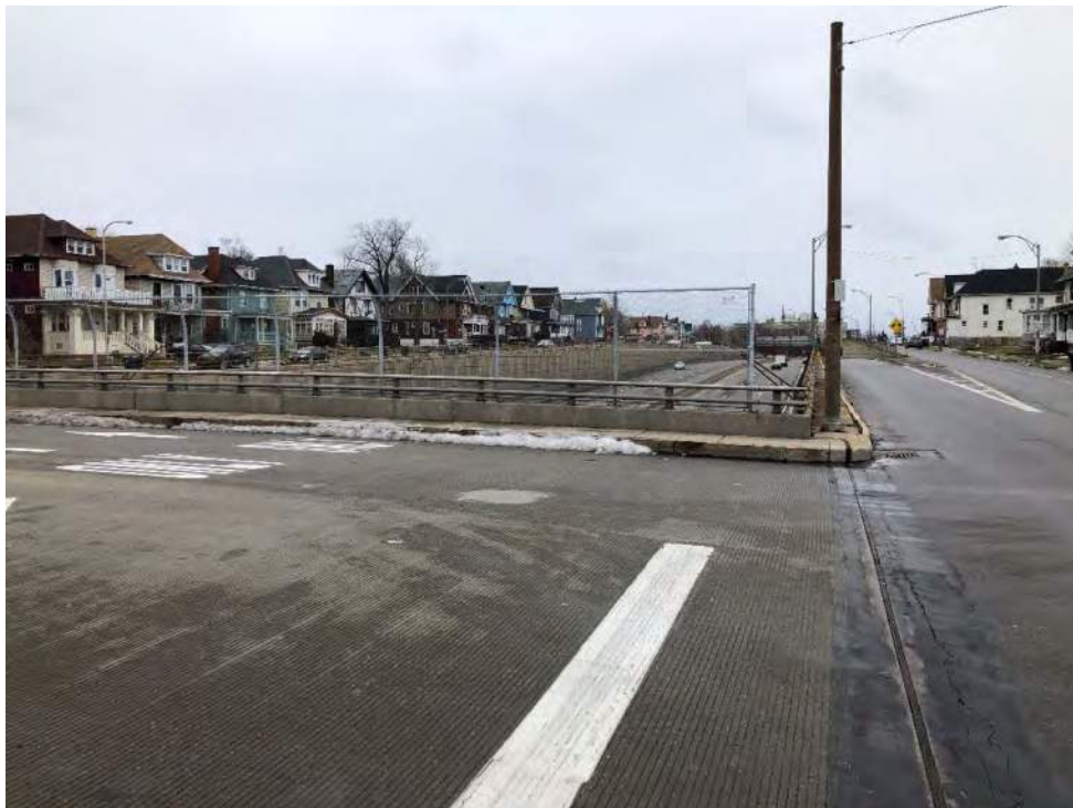
Photo 2 – View looking north at BIN 1022630 (E. Utica Street over Kensington Expressway (NY Route 33)).
